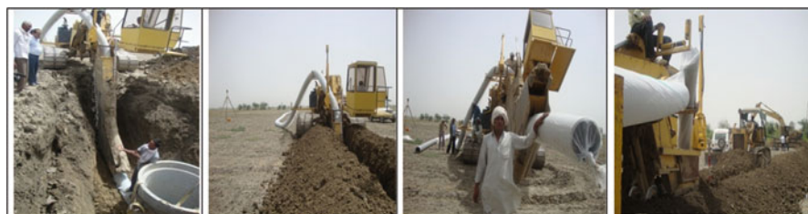
Fig. 18.5 Subsurface drainage machinery being used in Haryana
