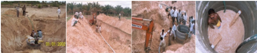
Fig. 18.9 Installation of radial collector Doruvu wells at Bapatla (Andhra Pradesh), India
