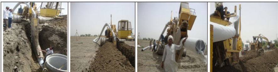
Fig. 18.5 Subsurface drainage machinery being used in Haryana
