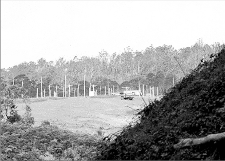
Fig. 21 The Hornsby Valley field station. (Courtesy: CRAIA)
