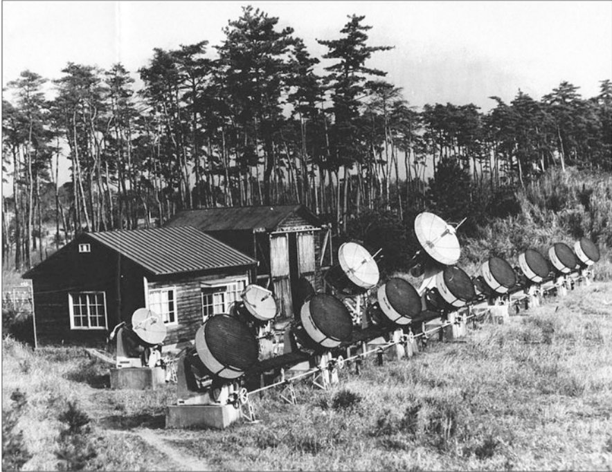
Fig. 46 The expanded 8-element solar grating array, complete with polarisation screens, and behind it the four total power radiometers that monitored the Sun at 1, 2, 3.75 and 9.4 GHz. (Courtesy: Tanaka Family)
