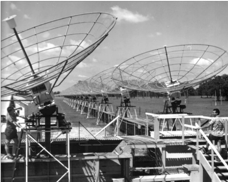
Fig. 36 A view looking south along the N-S arm of the Chris Cross from near the centre of the array. (Courtesy: CRAIA)
