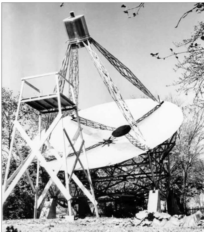
Fig. 5 Reber's 32-ft (9.75-m) parabolic antenna built at Wheaton in 1937. (Courtesy: National Radio Astronomy Observatory)
