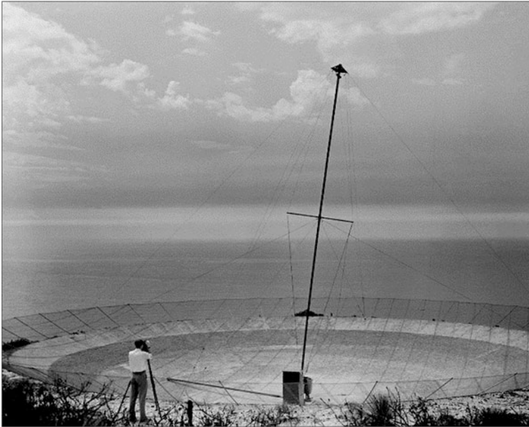
Fig. 19 The 80-ft ‘hole-in-the-ground’ antenna at Dover Heights. Gordon Stanley is using a theodolite to record the tilt of the aerial mast. (Courtesy: CRAIA)
