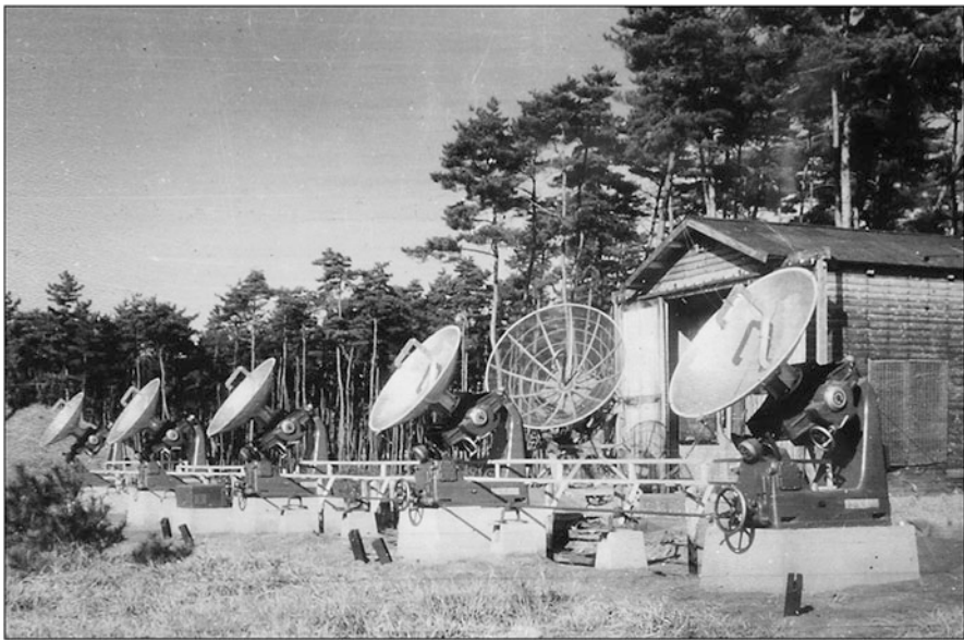
Fig. 45 The 5-element E-W grating interferometer in 1953, with the original Toyokawa antenna in the background. (Courtesy: Tanaka Family)
