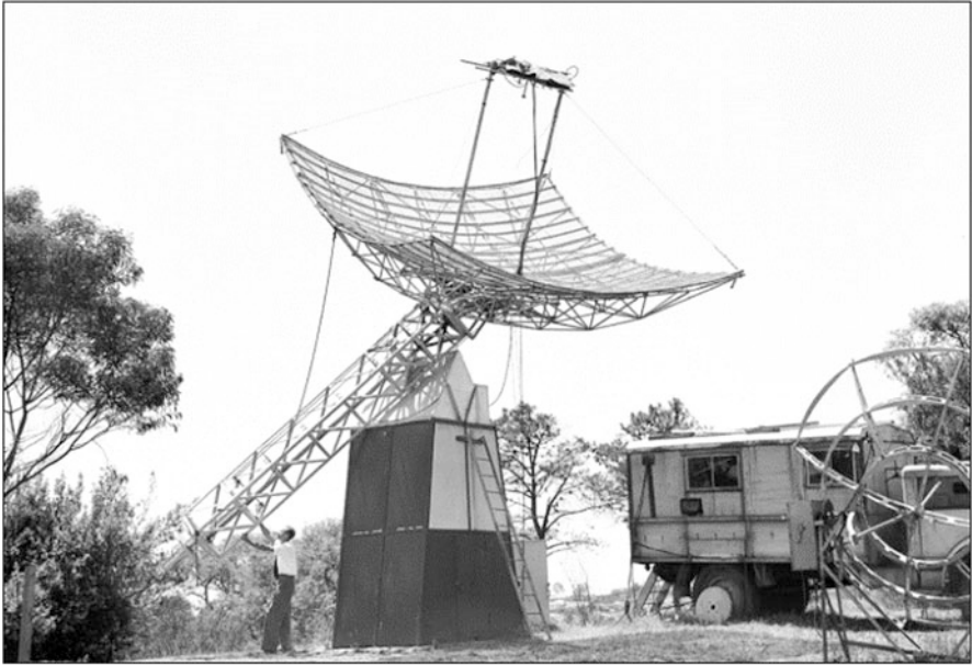
Fig. 28 This antenna was originally at RP's Georges Heights field station, and had started life as an experimental radar aerial. At Georges Heights it was modified for radio astronomy and used for solar observations at 600 MHz and 1.2 GHz. In 1948 it was transferred to Potts Hill in time for the 1 November solar eclipse, and then was used by Piddington and Minnett for their all-sky surveys before serving as the initial H-line antenna. (Courtesy: CRAIA)
