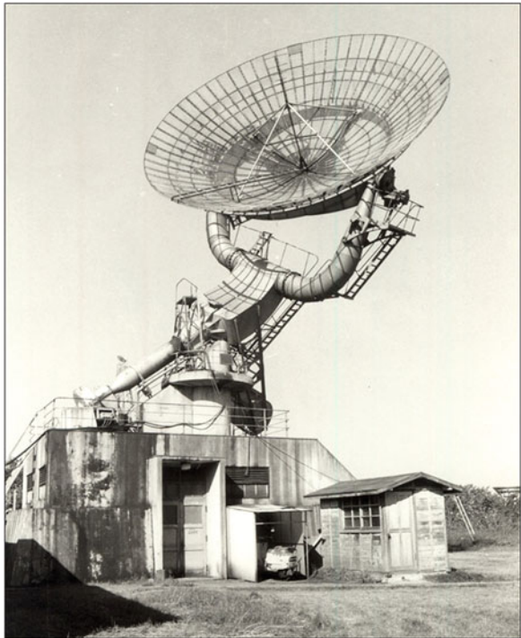
Fig. 43 This 10-m parabolic radio telescope installed in 1953 was used for solar monitoring at 200 MHz and 3 GHz. (Courtesy: NAOJA)
