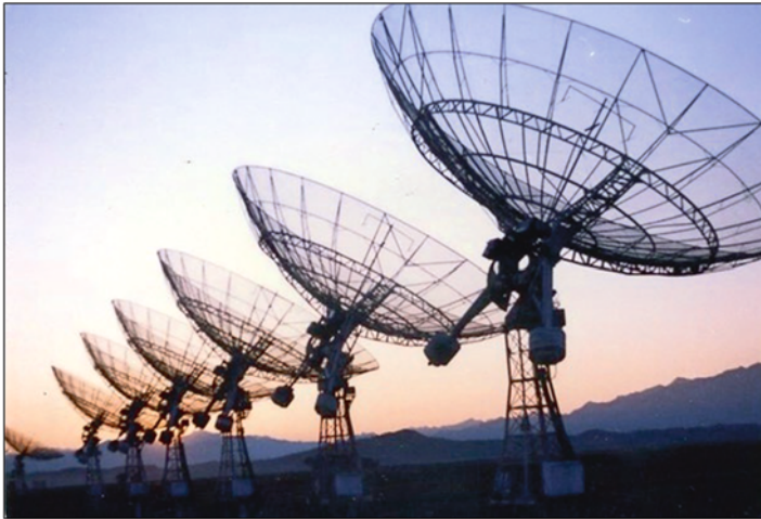
Fig. 63 The Miyun 28-element Meter Wave Aperture Synthesis Array. (Courtesy: Beijing Astronomical Observatory)
