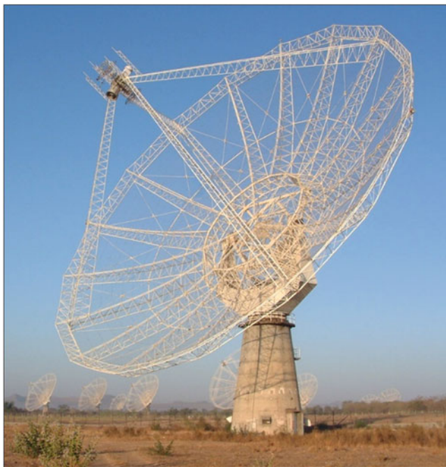
Fig. 58 A close up of one of the 45-m antennas, with eight others in the background. (Courtesy: TIFR archives)
