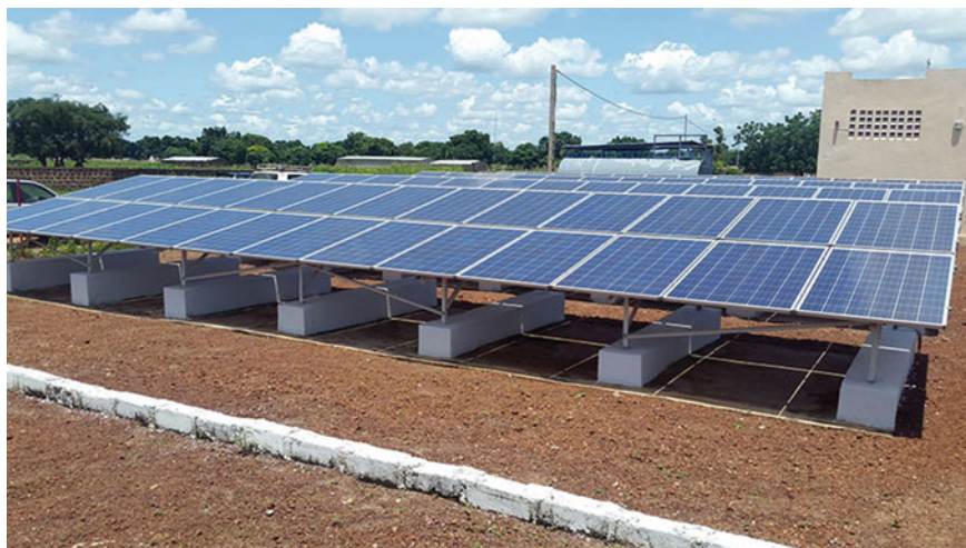
Fig. 7.12 Solar field in NIENA, Rural locality have benefited from a hybrid system (solar photovoltaic/diesel). This plant provides electricity to 538 customers. Installed power: 100 kva, Solar power: 50 kw. Source World Bank 2017
