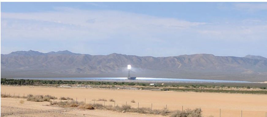
Fig. 11.1 Photograph of one of the power towers and heliostat fields of the Ivanpah solar thermal power plant in the Mojave Desert in California at the border with Nevada. Photo credit V. Narayanan
