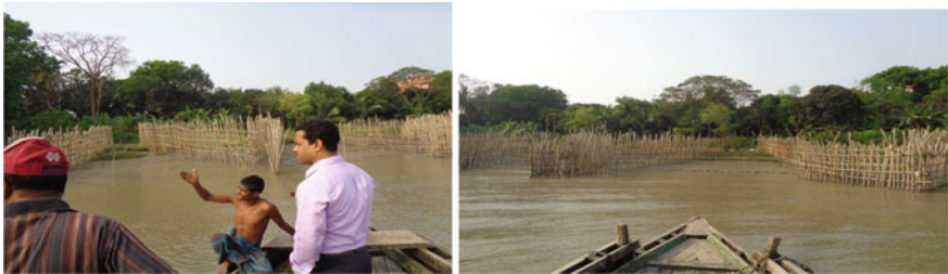
Fig. 9 The river bank of Rupsha River is protected by using bamboo bandalling structures at Khulna, Bangladesh
