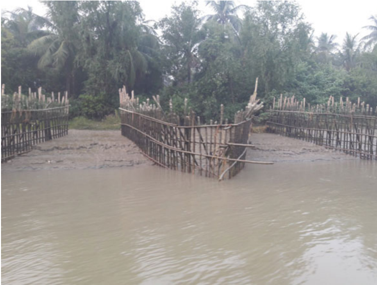
Fig. 10 Photographs shows the sediment deposited near the eroded bank within the bamboo bandals field
