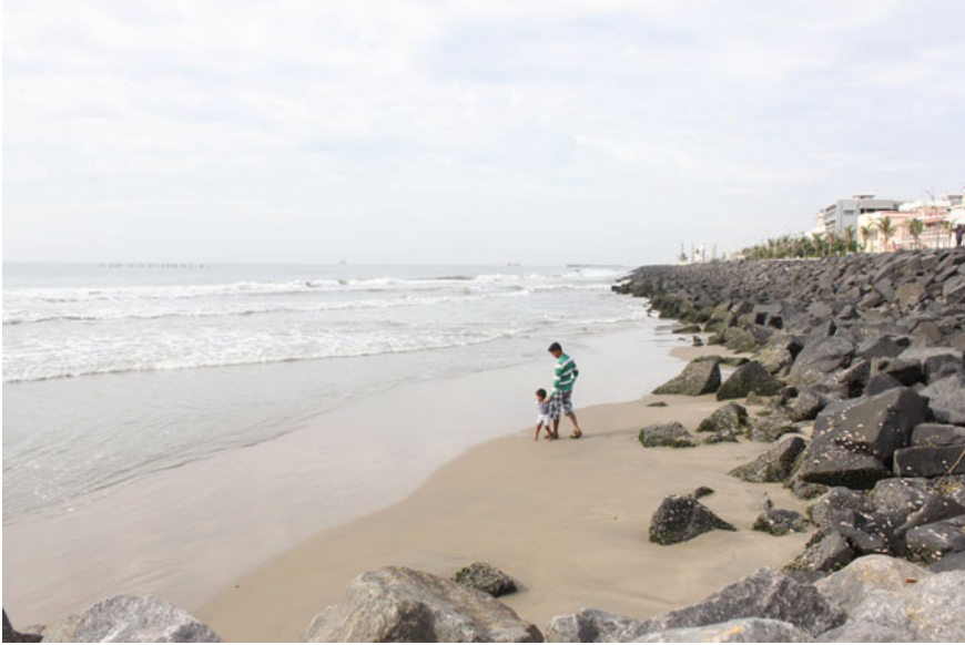
Fig. 1 Beach eroded away
