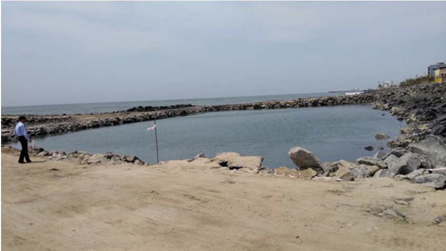
Fig. 11 Progressing with the work area
