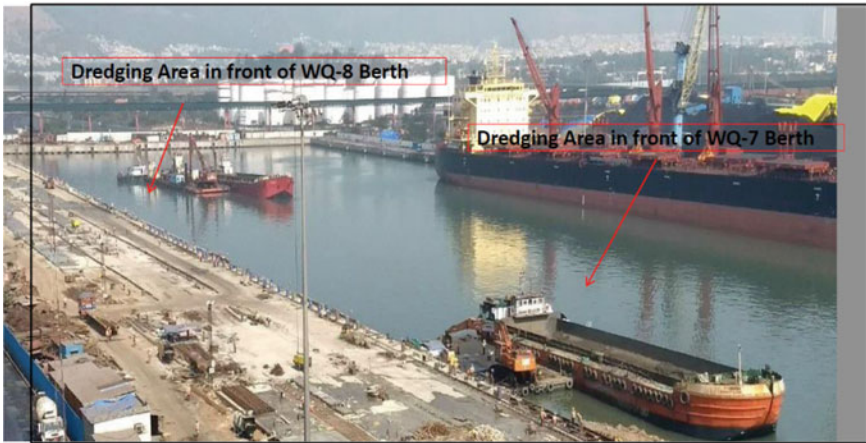
Fig. 2 Dredging work in Vizag Port
