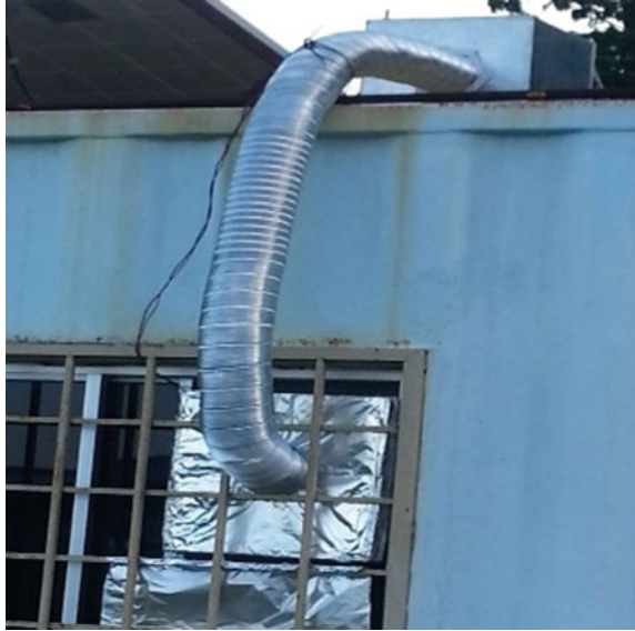
Fig. 6 Assembly of the ducting pipe to the exhaust fan
