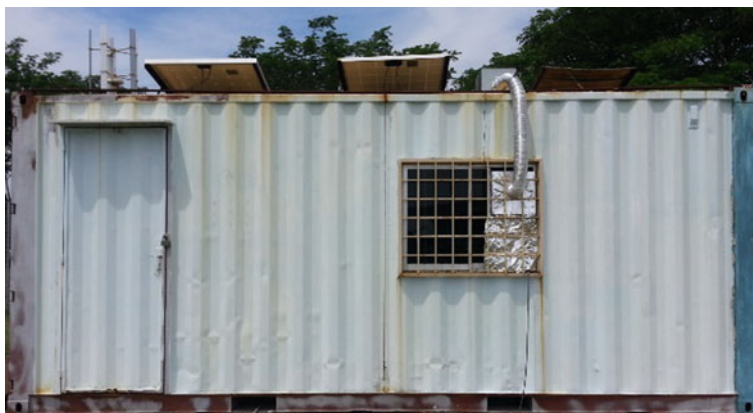
Fig. 8 Final product of the solar-powered ventilation system
