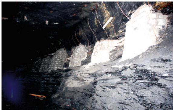
Fig. 5 Pillar sides supported with fly ash bricks
