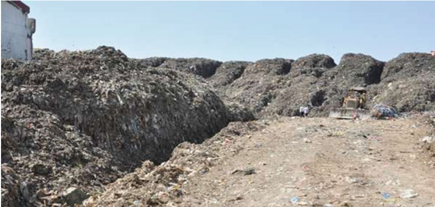
Photo 7 Huge windrows formed by slicing and trenching brought down the heap height
