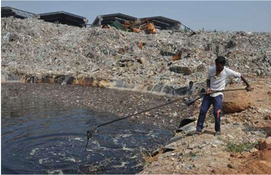
Photo 3 Waste floating on leachate pools was removed manually with rakes
