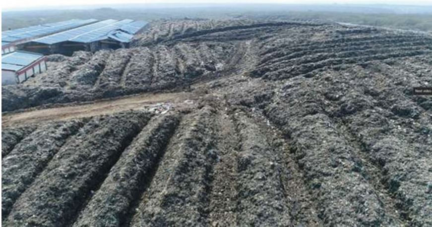
Photo 9 All old plus fresh waste bioremediated in windrows, ready for biomining
