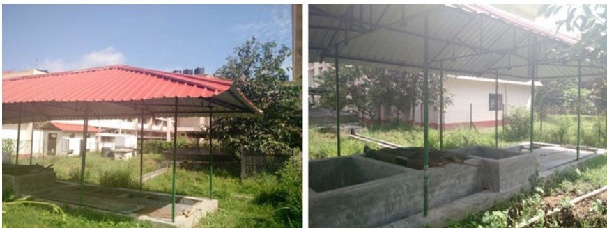
Fig. 3 Separation of digestate and its conversion to vermicompost
