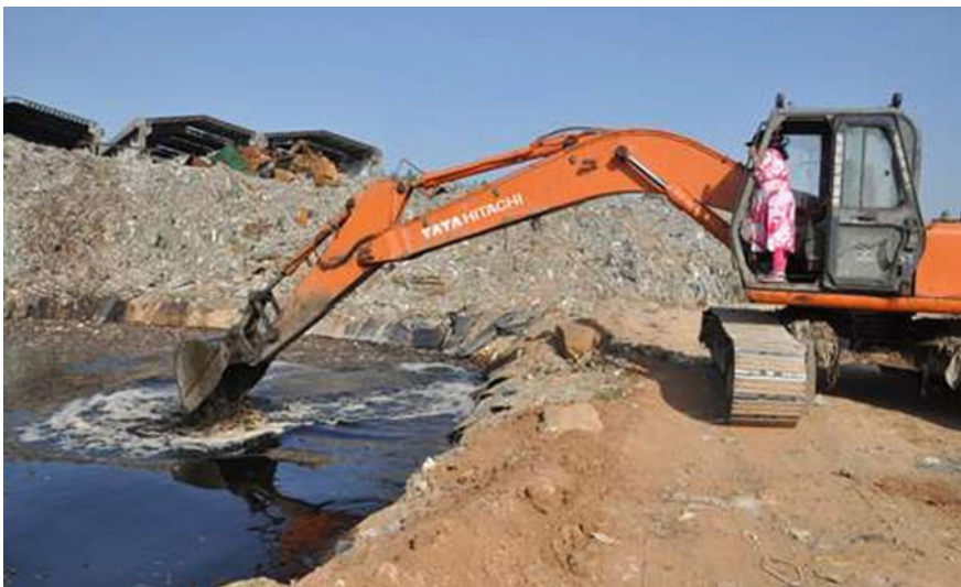
Photo 4 Leachate pool aeration using a JCB bucket
