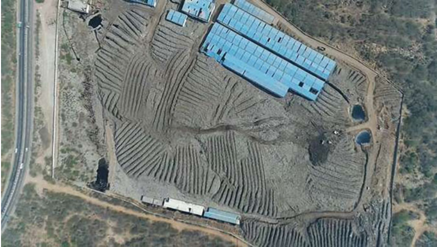
Photo 11 By December 2017, nearly 95% percent of the original leachate present had been drained out and digested, with leachate present in only in a few small pools
