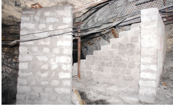
Fig. 3 Masonry roof support with fly ash bricks
