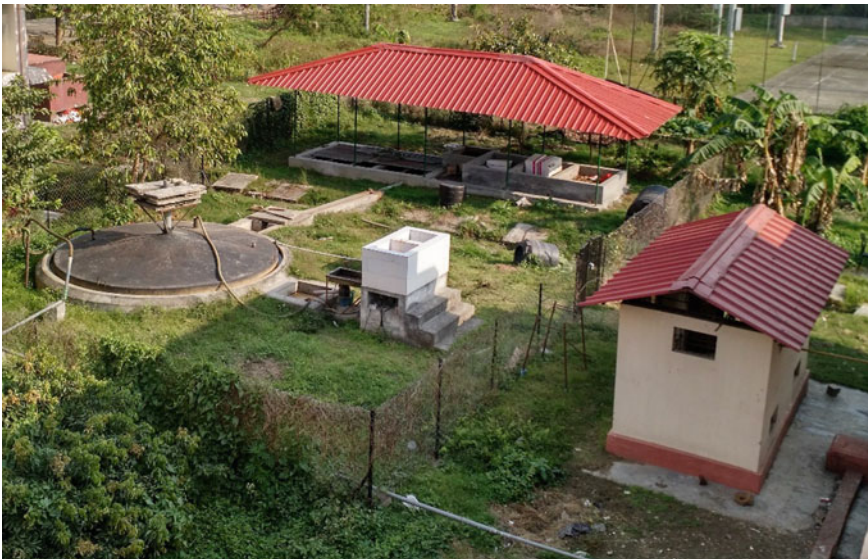
Fig. 1 Complete kitchen-waste-fed biogas plant with slurry handling and vermicomposting unit
