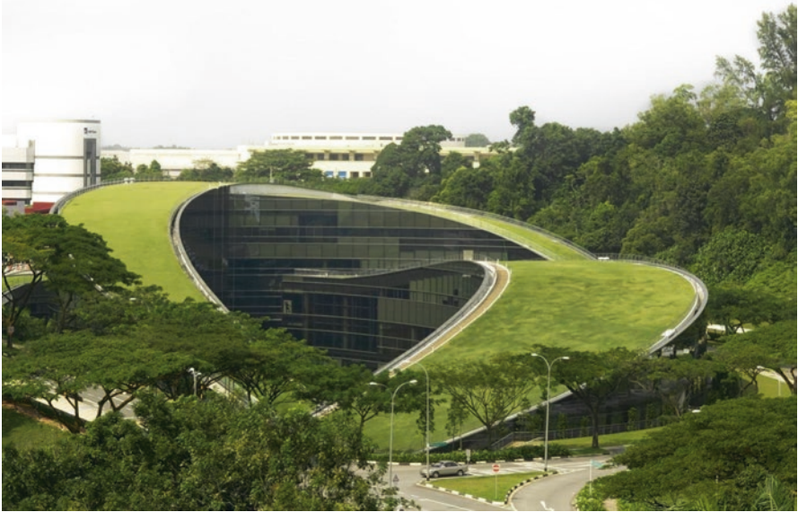
Fig. 1.5 Extensive green roof on School of Art, Design & Media at NTU, Singapore
