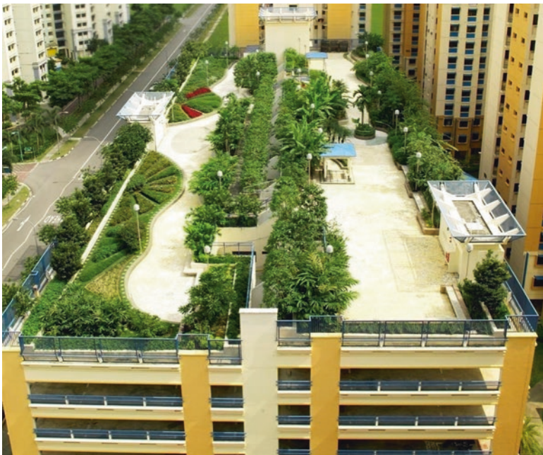
Fig. 1.6 Intensive green roof on parking structure, Singapore
