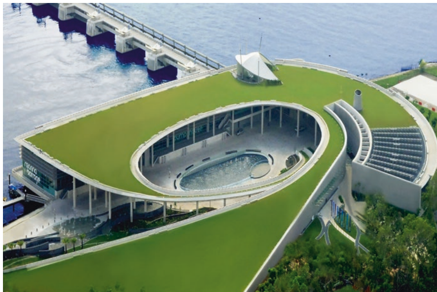
Fig. 1.3 Singapore marina barrage reservoir
