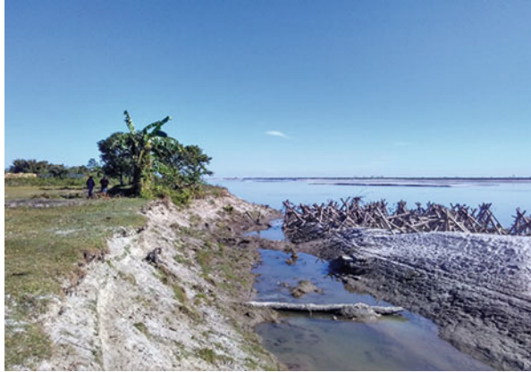
Plate 5 RCC porcupines for bank strengthening on R. Lali
