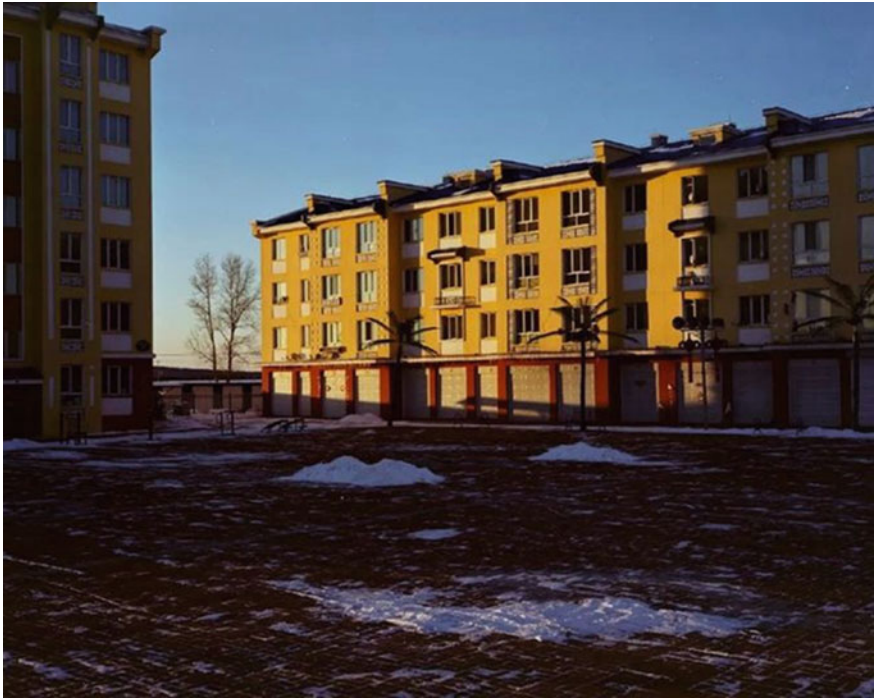
Fig. 12.10 A mostly abandoned residential building in Yichun, which is suffering from the structural crisis
