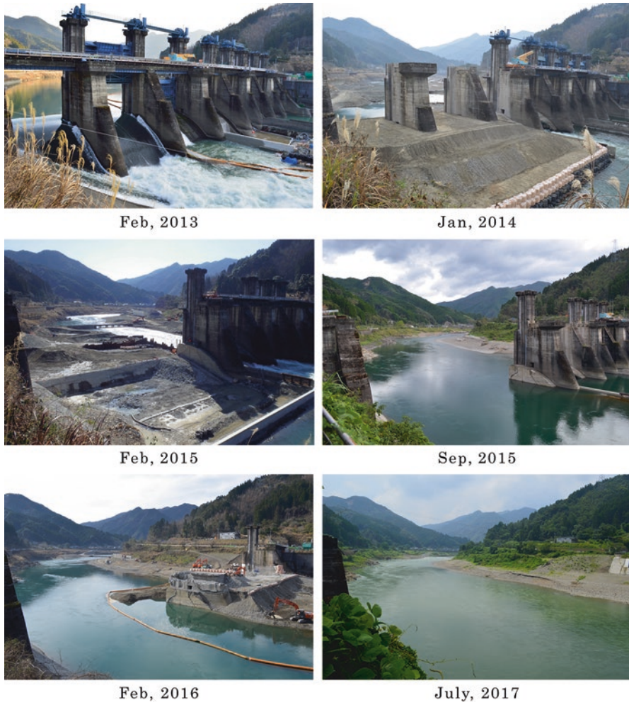
Fig. 3.4 Progress of the Arase Dam removal work
