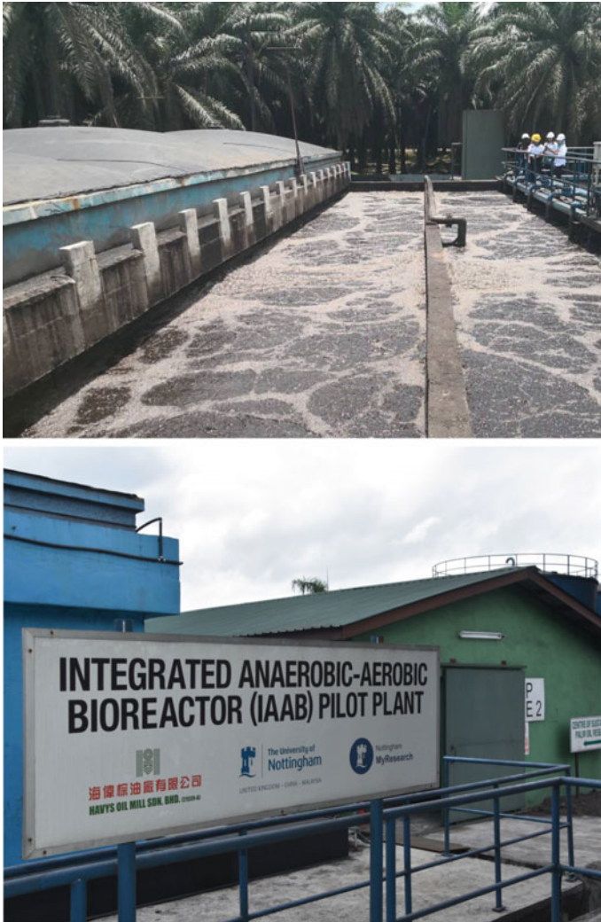
Fig. 9 Pre-commercialised scale of IAAB system (courtesy of Havys Oil Mill Sdn. Bhd.)
