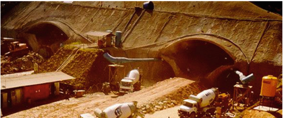
Fig. 3. External and internal tracks of “São Paulo Rodoanel Highway” [2]
