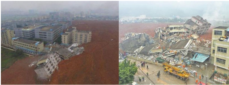
Fig. 2. Some damaged buildings on site
