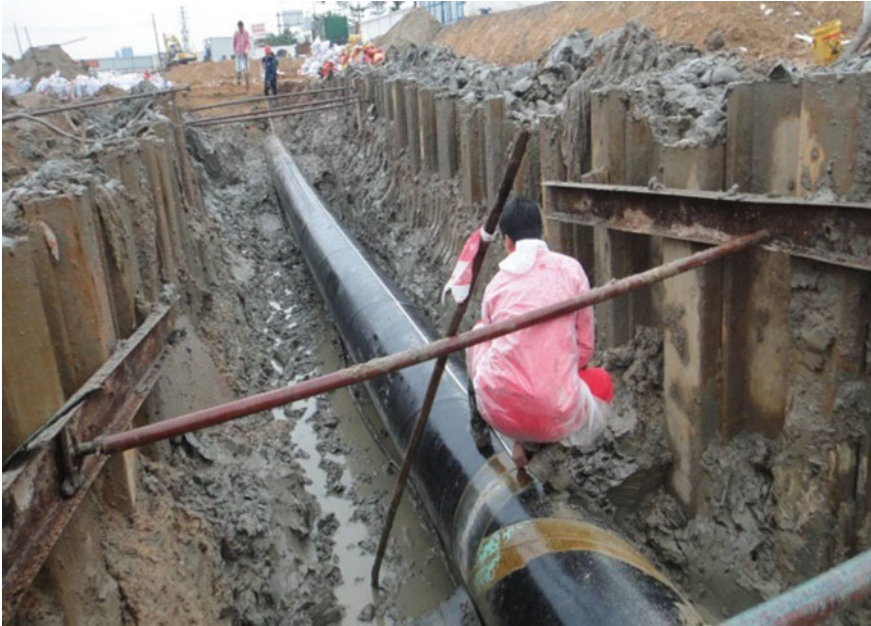
Fig. 2. Excavation picture of slip pipe
