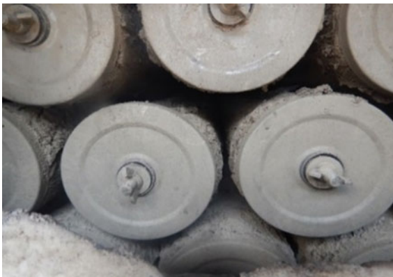
Fig. 4. Solids (mainly sulfur) in separator filters
