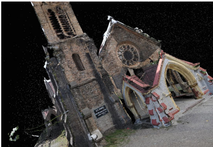
Fig. 19.8 Resultant point cloud of church after geo-registration
