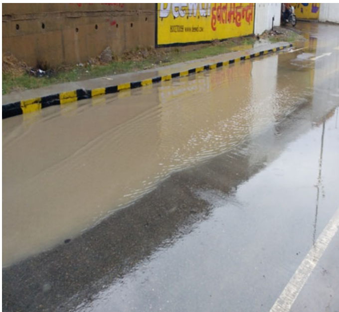
Fig. 6 Stagnation of water during rainy seasons
