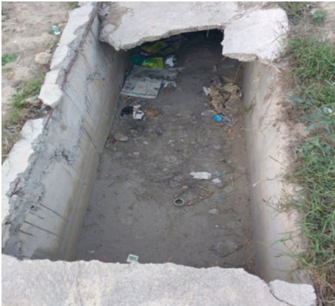
Fig. 1 Uncovered drain
