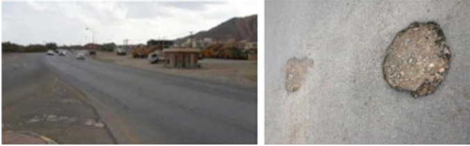
Fig. 1 Izki road, Muscat (Oman) and distress (Pothole) shown on the road [22]
