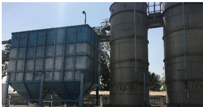
Fig. 2 Fluidized aerobic bio-reactor I and II
