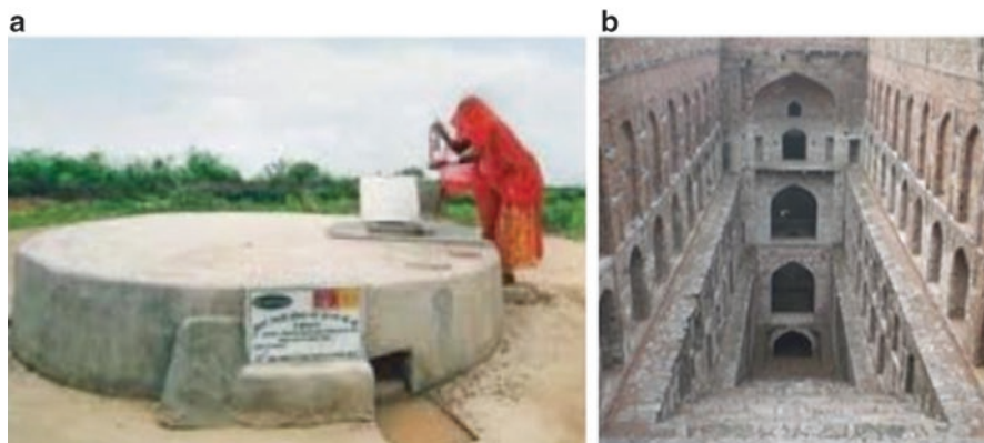
Fig. 3 (a) Tanka or underground storage of rainwater, (b) Baolis or stepwells for groundwater recharge and development
