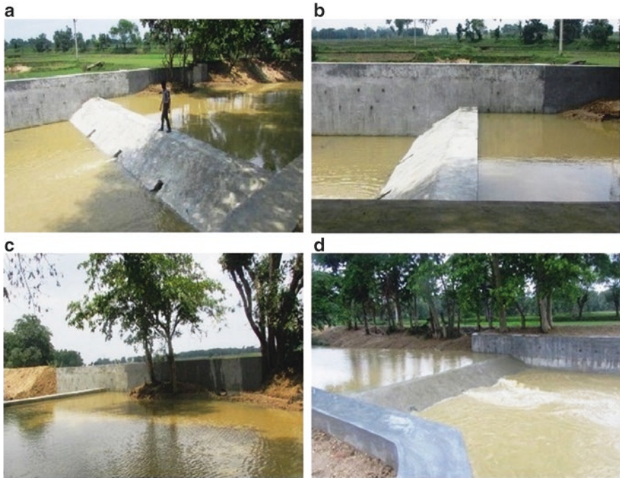
Fig. 8 (a–d) Synoptic view of check dam
