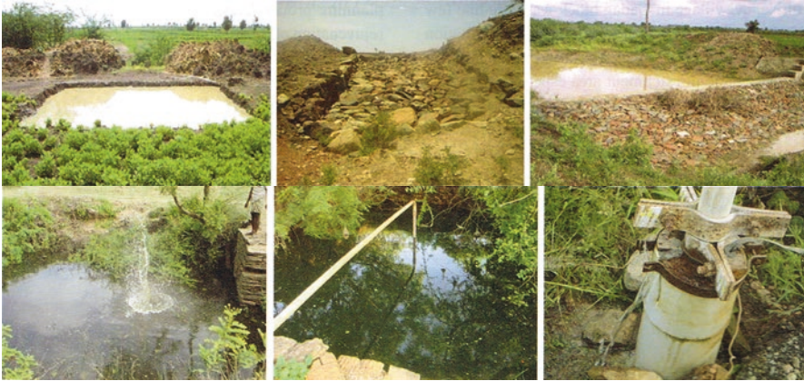
Fig. 4 Top row: (a) Rain water harvesting structures: farm ponds and stone checks across primary streams in Ichalahalla watershed. Bottom row: (b) Rejuvenation of open wells and bore wells in Ichalahalla watershed. (Source: Hiregoudar et al. 2016)
