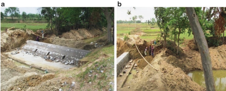
Fig. 7 (a, b) Construction phase of check dam of the study area
