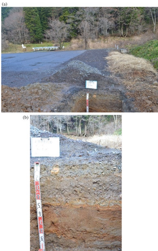
Fig. 13.3 Overview (a) and soil profile (b) of Parking lot
