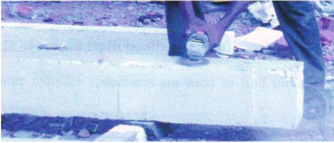
Fig. 3 Grinding the tension face of beam
