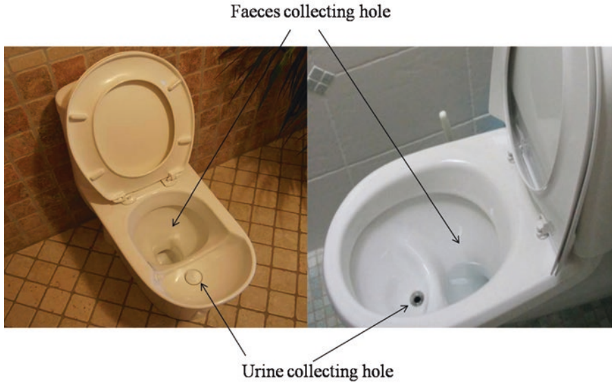
Fig. 9.11 Dry urine-diverting toilets
