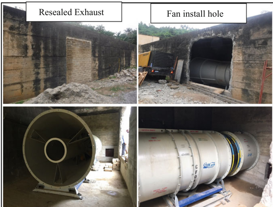
Fig. 9. Photos of main fan installation
