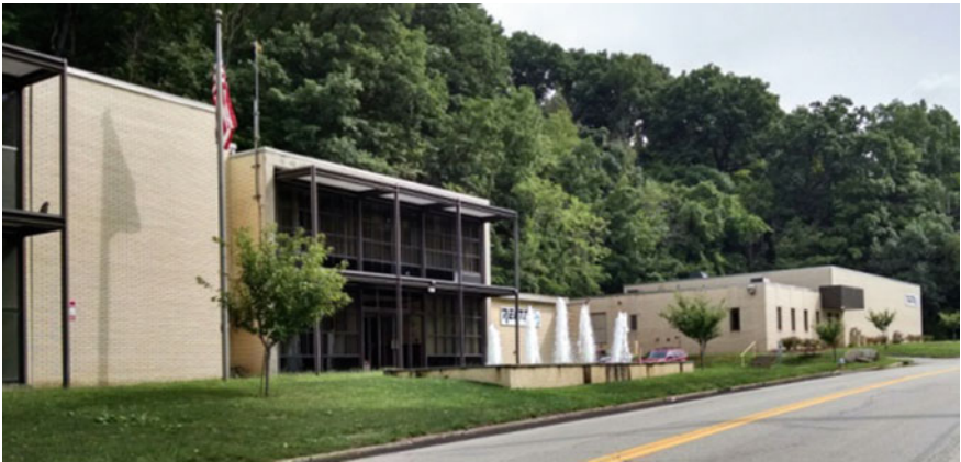
Fig. 8. Rel-Tek safety technology center
