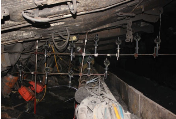
Fig. 1. Measuring system to analyse the distributions of air velocity and methane concentration fields
