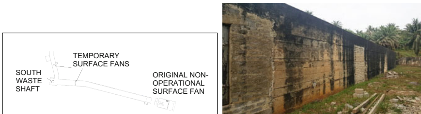
Fig. 5. Surface concrete tunnel with temporary fans shown
