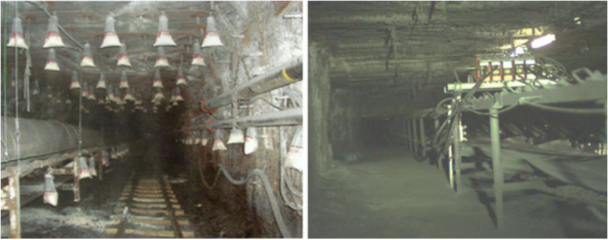
Fig. 4. Examples of a passive (left) and an active (right) barrier configuration to ensure obstacle coverage
