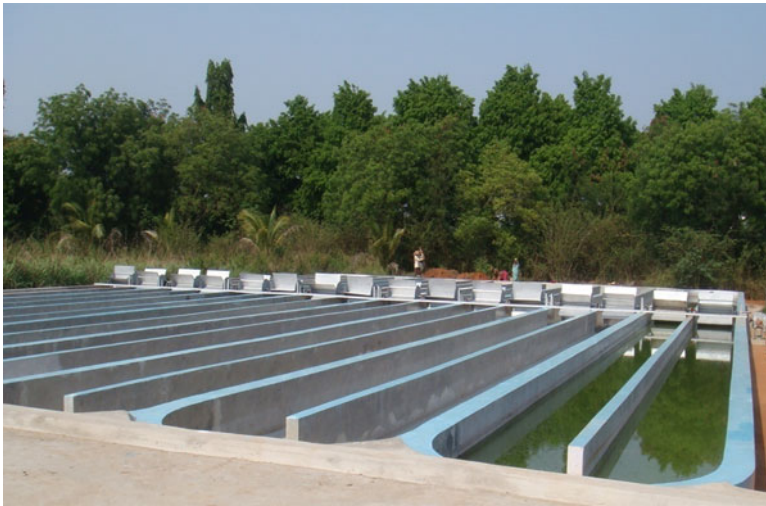
Fig. 12.3 Large-scale microalgae cultivation facility at CSIR-IMMT, Bhubaneswar, Odisha, India. Eight raceway ponds fitted with paddle wheels and CO 2 supply system
