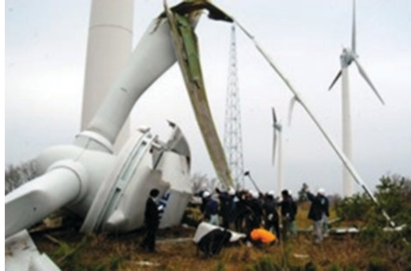
Fig. 5.2 Serious accident in a wind turbine
