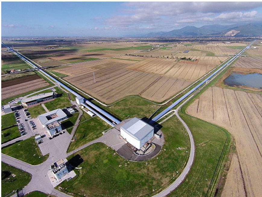
Fig. 12.6 Aerial view of the interferometer detector Virgo (Cascina, Pisa, Italy). From the Virgo collaboration under the Creative Commons CC0 1.0 Universal Public Domain Dedication
