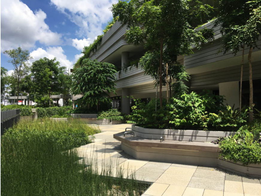
Fig. 9.4 Vegetative storm water filter, Kampung Admiralty, Singapore; Credit to Ramboll Studio Dreiseitl
