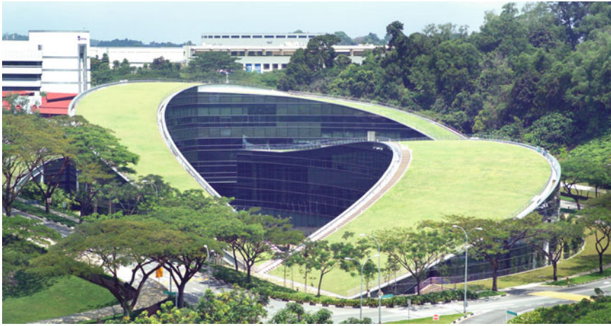
Fig. 12.1 Nanyang Technological University School of Art, Design and Media, Singapore; Credit to CPG Consultants
