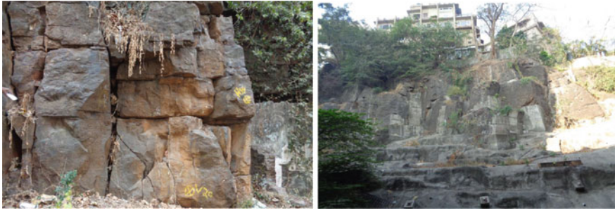
Fig. 1 Present rock slope appearance on out crops from eastern to western corner of the slope a dominant joint sets, discoloration, and staining of rock material due to weathering clearly visible b already stabilized portion of the rock slope
