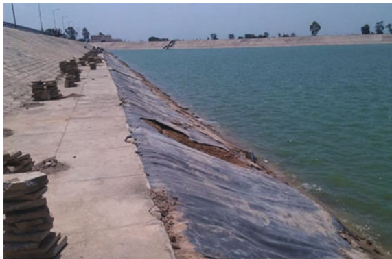
Fig. 7 Sliding of thin protection tiles over smooth geosynthetic laid over steep slopes
