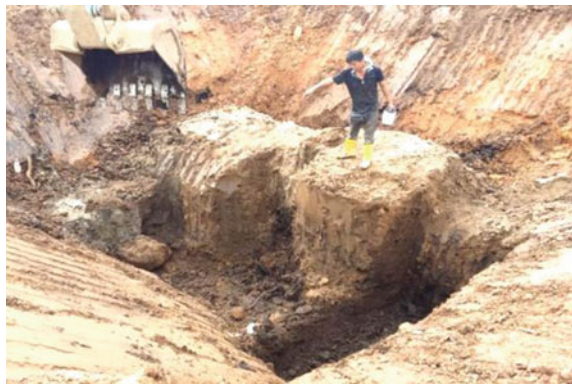
Fig. 11 Trench excavation shows successful formation of DSM piles in peaty soils
