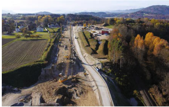
Fig. 13 Overview of Srejach Tunnel site
