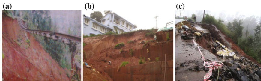
Fig. 9 View of case history sites; a slope failure at Aravankadu b retaining wall failure at Coonoor c slope failure at Chinnabikkaty (Chandrasekaran et al. 2013b)
