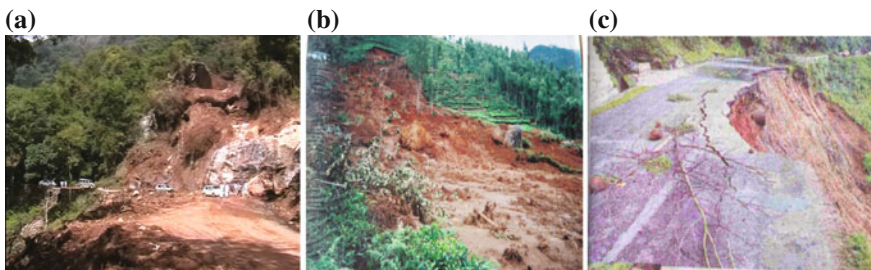
Fig. 10 View of landslides in Nilgiris; a Marappalam landslide b Achanakkal landslide c Madithorai landslide
