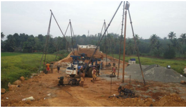
Fig. 9 Implementation of MFCI in bridge approaches at Gramenchira
