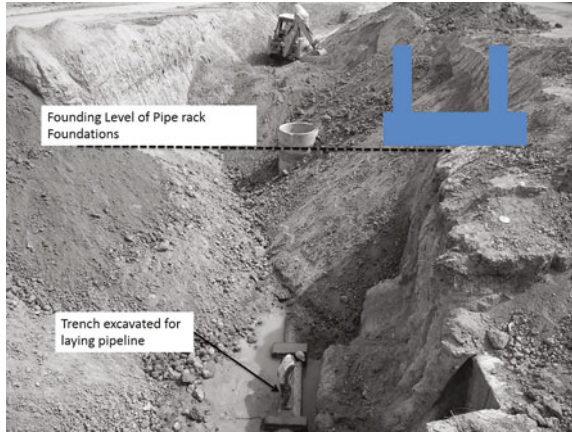
Fig. 11 The pipeline laying and backfilling relative to the pipe rack foundation
