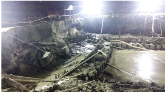
Condition of earth while excavated below RL (+) 1.45M
