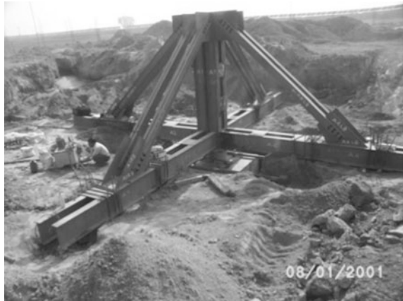
Fig. 2 Footing load test in progress
