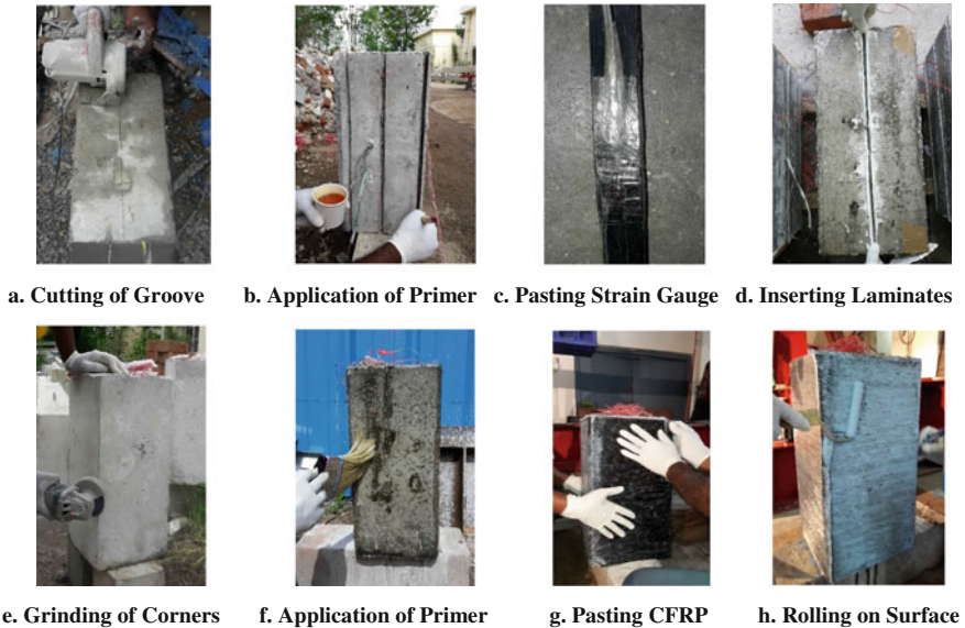
Fig. 2 a–h Strengthening of columns by hybrid strengthening technique
