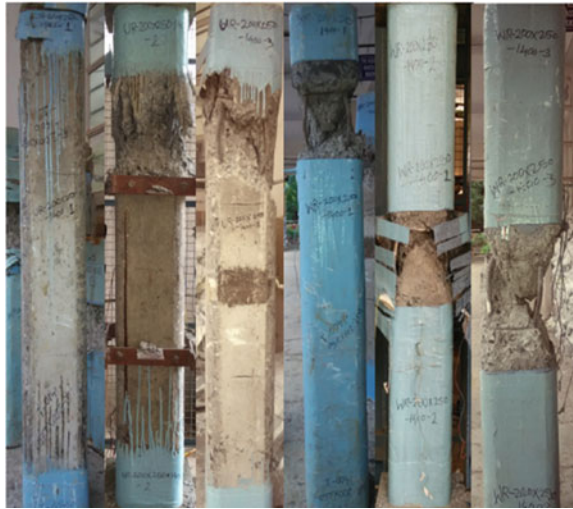
Fig. 3 Failure of unwrapped and wrapped columns, respectively (250 × 200, 1400)
