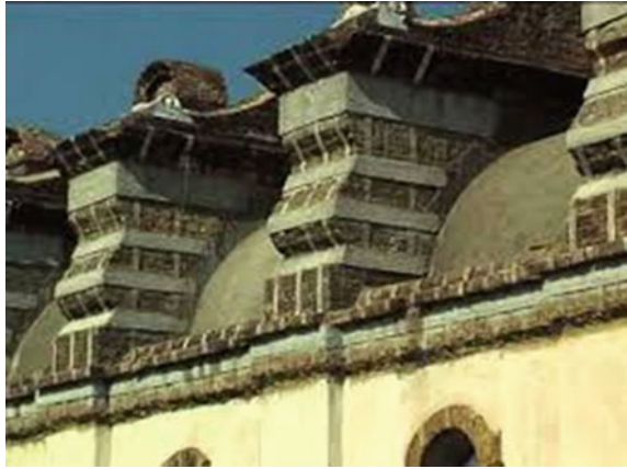
Fig. 9 Vertical reinforcement and horizontal GFRP wraps for masonry pier heads. Source http://english.cctv.com
