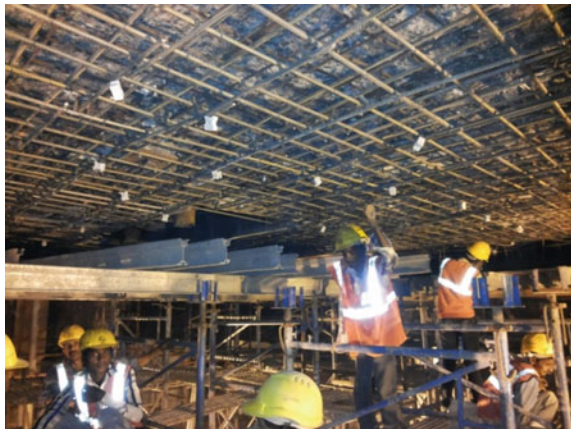
Fig. 15 Tying of reinforcement in progress (before concreting)
