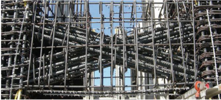
Fig. 1 Diagonal reinforcement detailing in coupling beam
