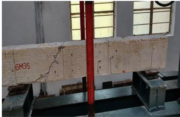
Typical crack pattern of shear beam Without fibres -6M3
