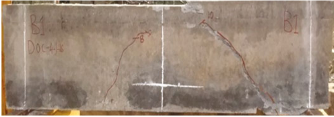
Fig. 3 Failure pattern of B1
