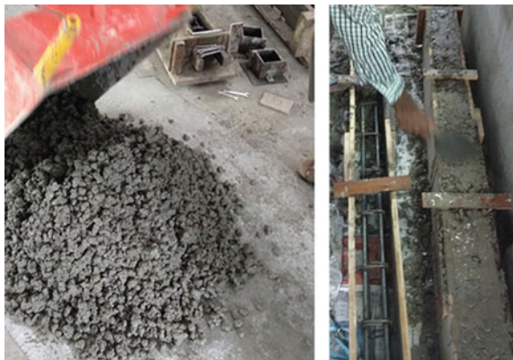
Fig. 4 Casting of typical geopolymer concrete beam
