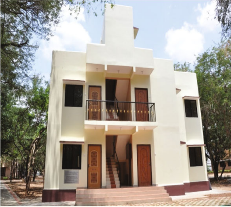
Fig. 3 GFRG demonstration building at IIT Madras campus
