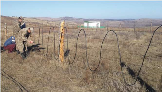
Fig. 4. Installation of sensor cable in the real field test
