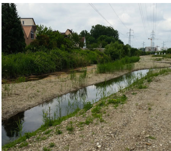
Fig. 3 Restored stream. A dead arm can be seen on the left side of the picture, and a meander on the right (Source ICube Laboratory)
