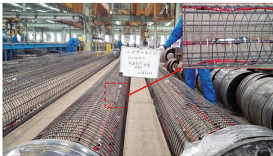
Fig. 3. Strain gauges installation
