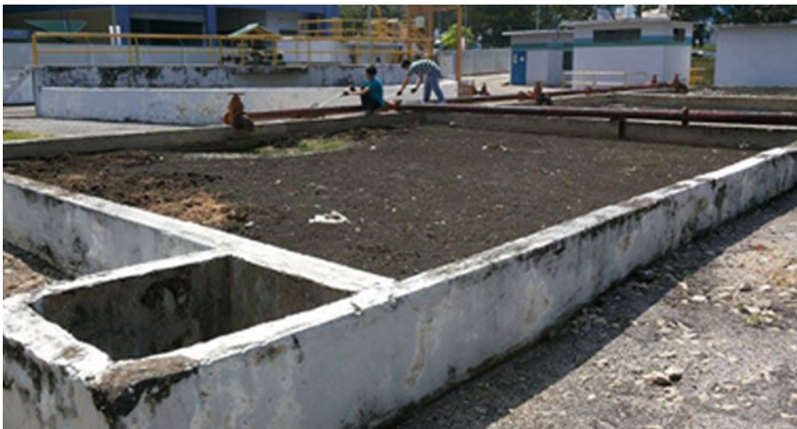
Fig. 1 Sewage sludge dried at the sludge bed under sun
