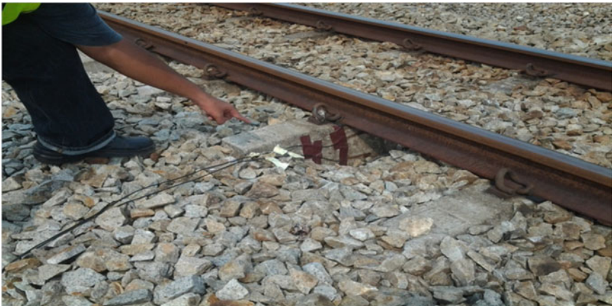
Fig. 2 Specimen was equipped with necessary gadgets
