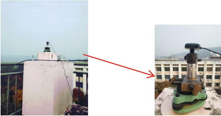
Fig. 6 Monitoring station CREF
