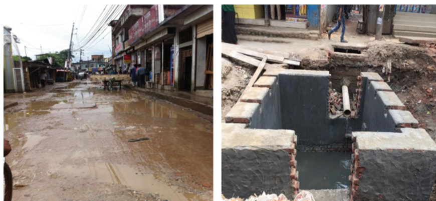
Fig. 8.7 Damage of roads and structures due to waterlogging in Dhaka city. Source Authors
