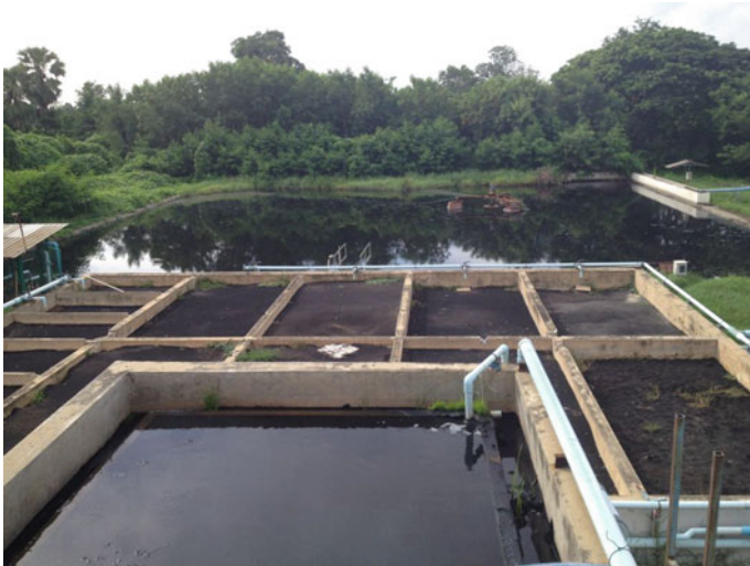
Fig. 6 Solar evaporation plant used in small-scale textile coloration units in Tirupur, India
