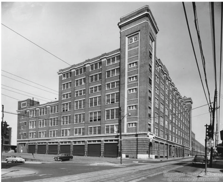
Historic shot of the Nabisco Factory, Bakery Square, Current Google Office. (Source: Historical Society of Western Pennsylvania)
