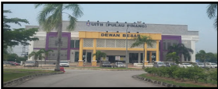
Fig. 1 Front view of UiTMPP's Dewan Besar
