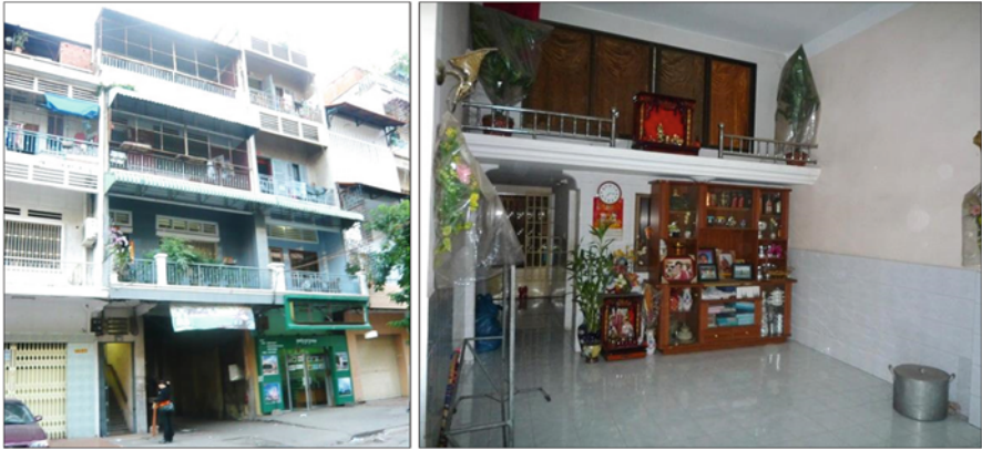
Fig. 41.6 Exterior (left) and interior (right) of the measured house
