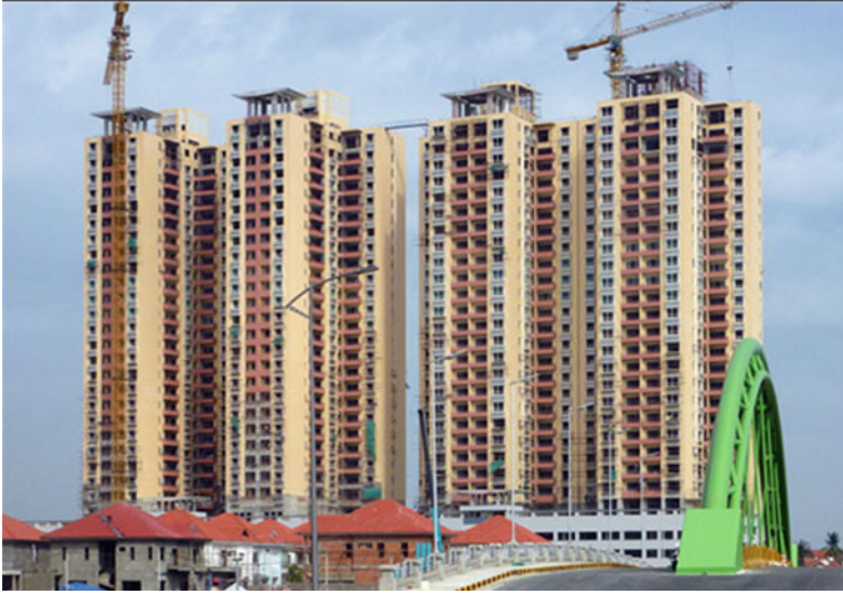
Fig. 31.4 Condominium (under construction)
