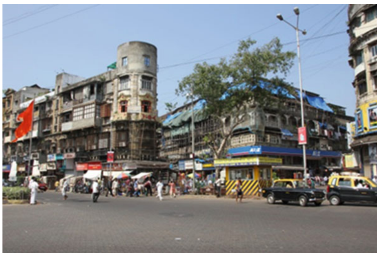
Fig. 16.1 A typical chawl of Mumbai with shops on the street front (Source: Marco Zanferrari)
