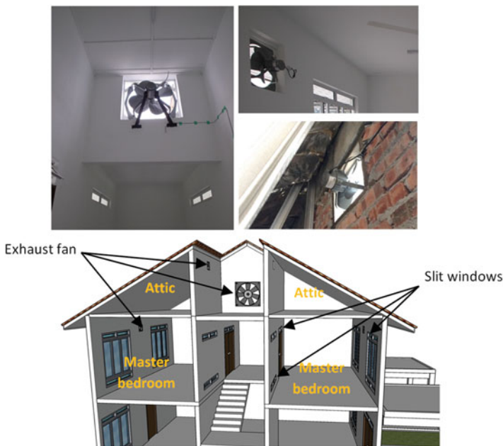
Fig. 43.2 Slit windows and exhaust fans employed in the experimental house
