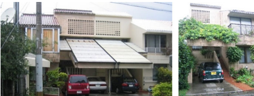
Fig. 46.5 Sueyoshi riverside house (Photo by Hirokazu Mitsuoka)
