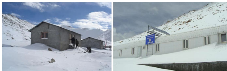
Fig. 32 Permafrost facility at Chang La with modern laboratories at a height of 17,600 ft AMSL
