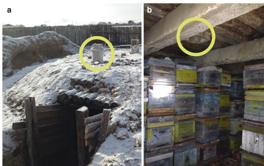
Fig. 9.5 Underground winter house for bees in condition of Mongolia. Circles show ventilation tubes. (a) Outside view, (b) inside view (Photo by Yondonjams G. Central region of Mongolia, November, 2014)
