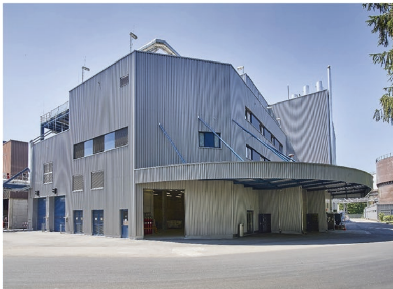
Fig. 10.5 New central sewage sludge treatment plant in Werdhölzli (Source: ERZ)
