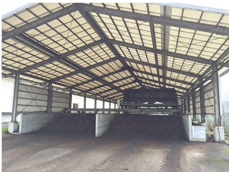
Fig. 25.1 Pile up aerobic fermentation
