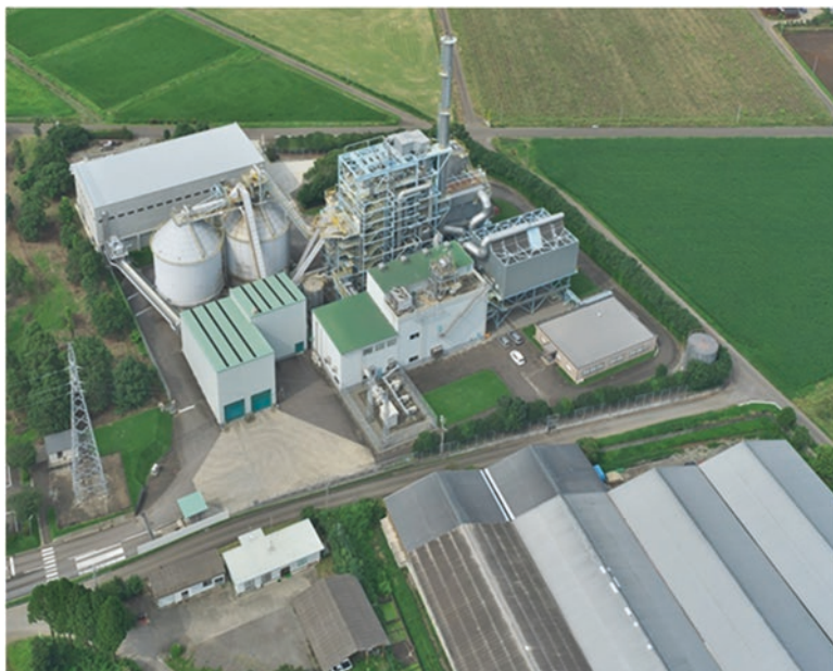
Fig. 1.6 Power plant for generating electricity by incinerating broiler chicken manure. (Photograph courtesy of K. Yano, MBR)
