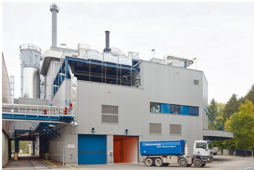
Fig. 15.2 Zürich Werdhölzli municipal sewage sludge incineration plant (Source Outotec)
