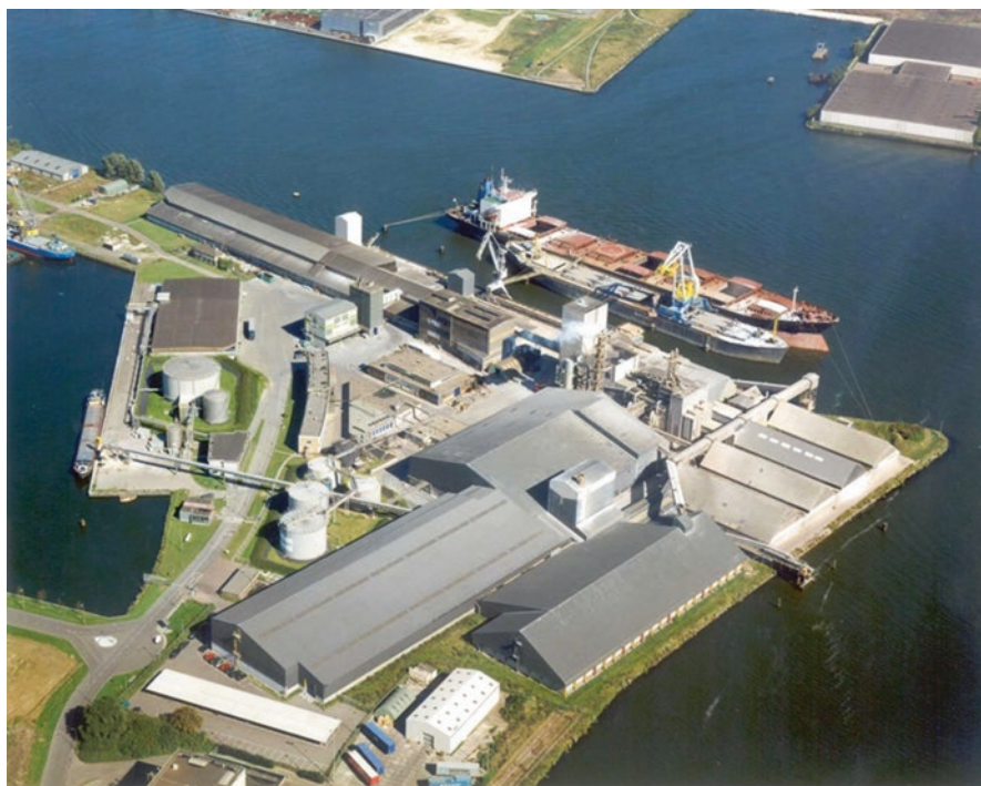
Fig. 16.1 ICL Fertilizers' production plant in Amsterdam
