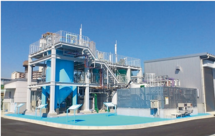
Fig. 17.7 The full-scale plant for struvite recovery plant at the Higashinada WWTP in Kobe, Japan
